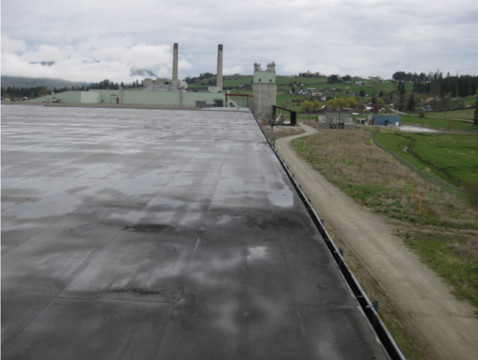
Existing Safety Condition
